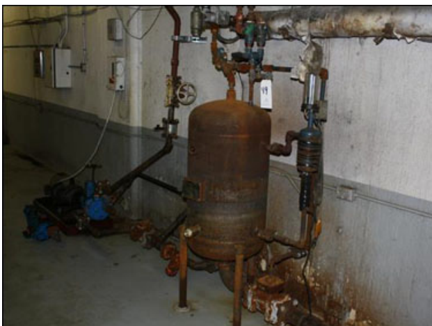
Picture taken prior to removal:
